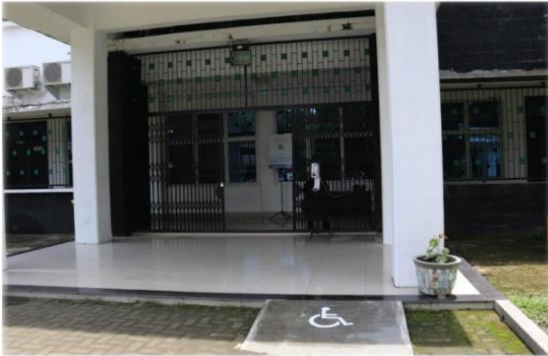
Facility for disability person using wheelchair on Faculty of Public Health
