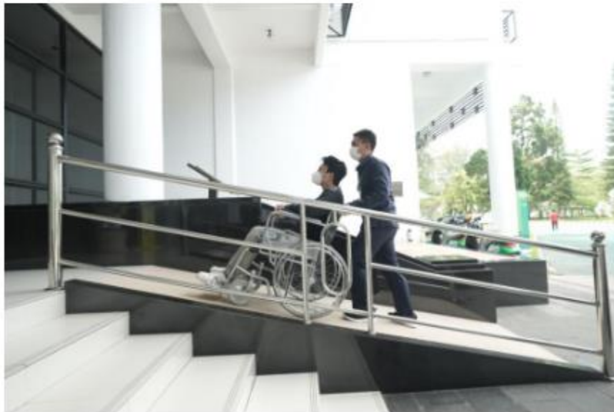
Road for disability person on Bureau Central Administration
